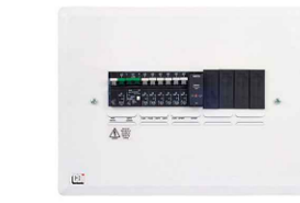
TYPICAL DISTRIBUTION BOARD
